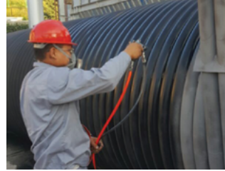
HiE-Coat™ 840-M coats industrial heat exchanger.
