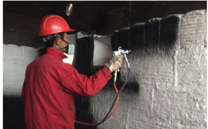
HiE-Coat™ 840-C applied to ceramic fiber module.
