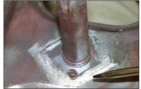
Pyro-Putty® 653 seals corroded burner manifold.
